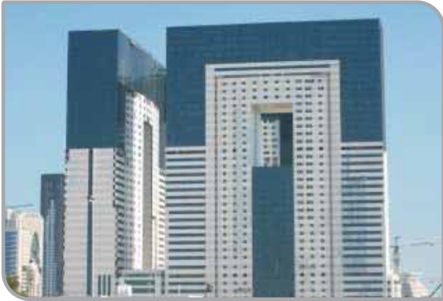
Dafna Tower 3&4, Doha
